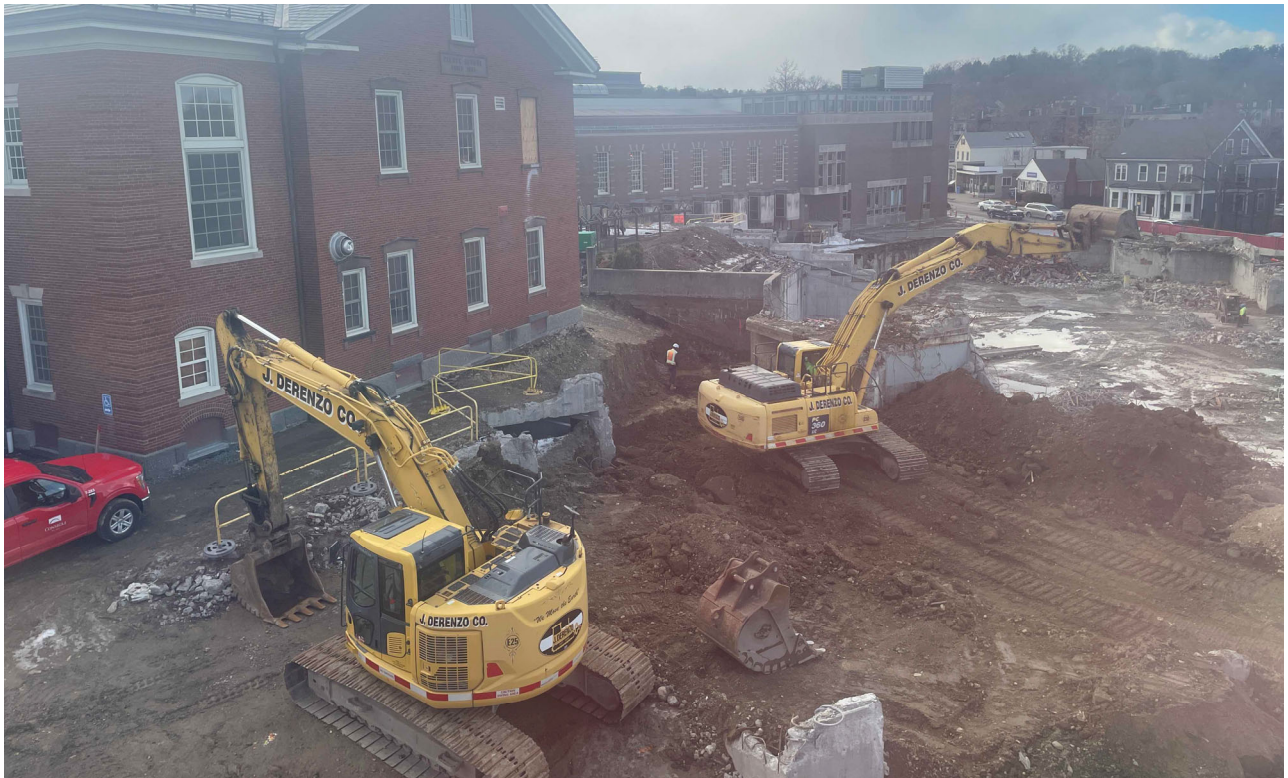
Work adjacent to Historic Building for pile installation.
