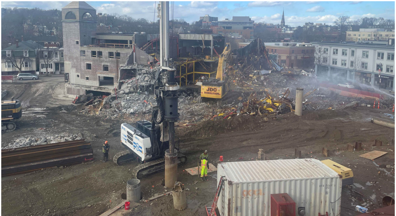
Pile drilling/installation.
